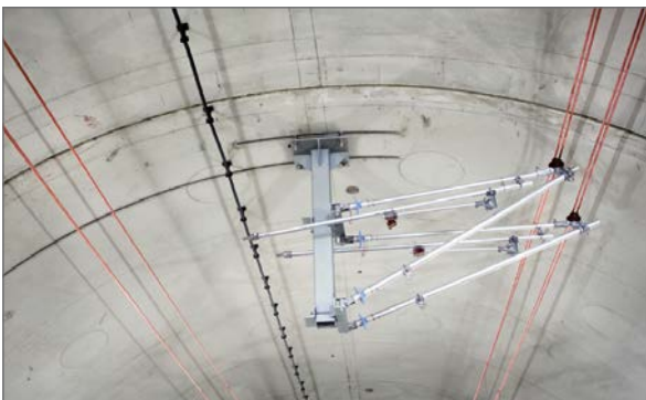
Curved anchor channels are used around the world to fasten overhead lines in railway tunnels.
