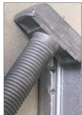
The notched teeth of the T-bolt are pressed into the channel lips.
