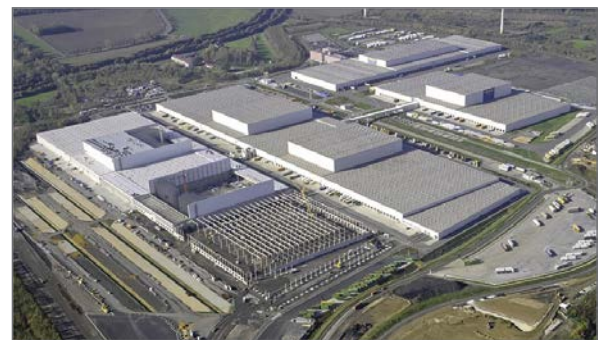
Installed on roof.
