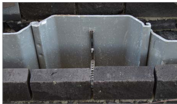
Connection of brickwork to sheet-pile wall.
